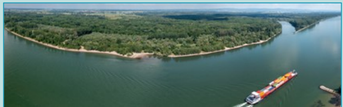
Picture 2: Restored riverbanks along Germany's federal waterways (Source: BfG).
