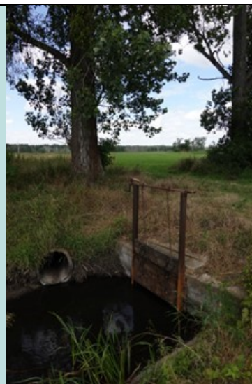
Picture 2.1: (a) project site with extensive grassland, (b) weir regulating the periodic flooding and re-wetting of the grassland (Source: Marie-Isabell Lenz, BfG, July 2024).
