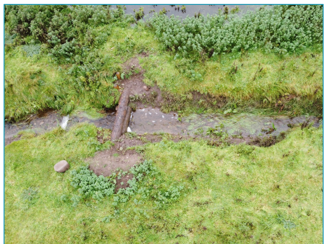
Figures 5 and 6: Two leaky dams with channel and pond (left), and single leaky dam measure (right) at the Forth Catchment (photos by Forth Rivers Trust)
