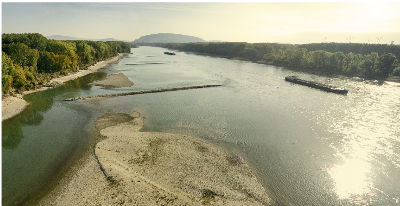
Figure 15 Instead of eight traditional groynes, only four innovative groynes regulate the Petronell-Witzelsdorf ford. They were combined with bank restoration. The picture shows the situation with low water. © viadonau/Zinner
