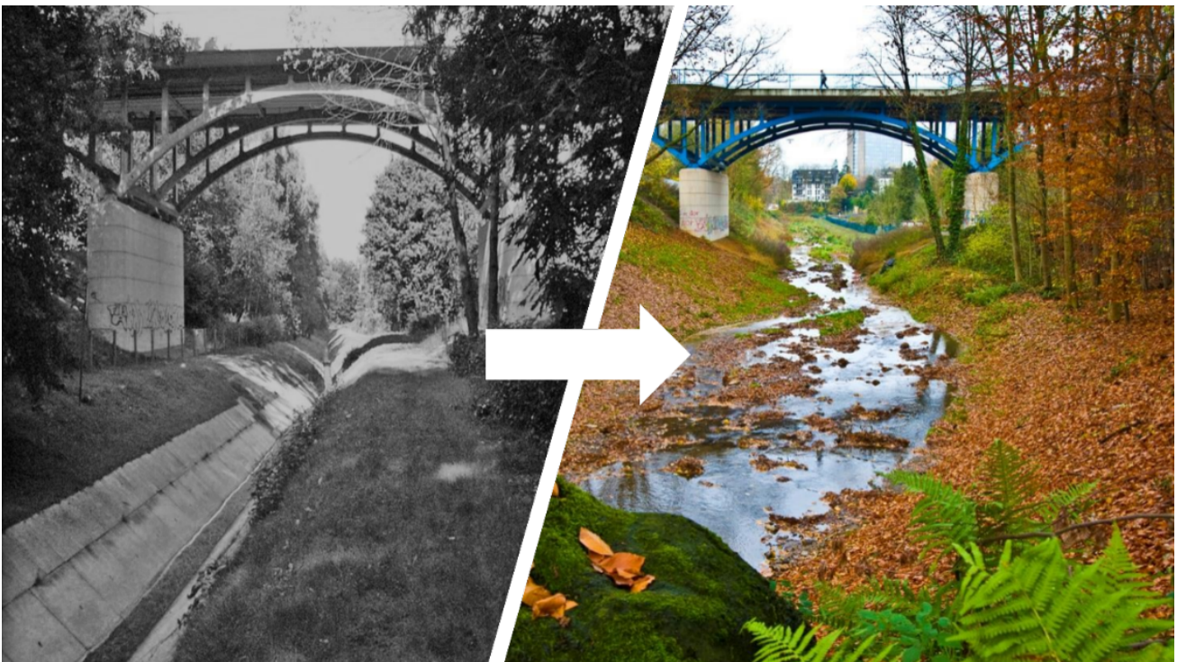
Figure 10: Revitalised stream (Borbecker Mühlenbach) as an example for the successful restoration of the smaller tributaries in the Emscher catchment area
