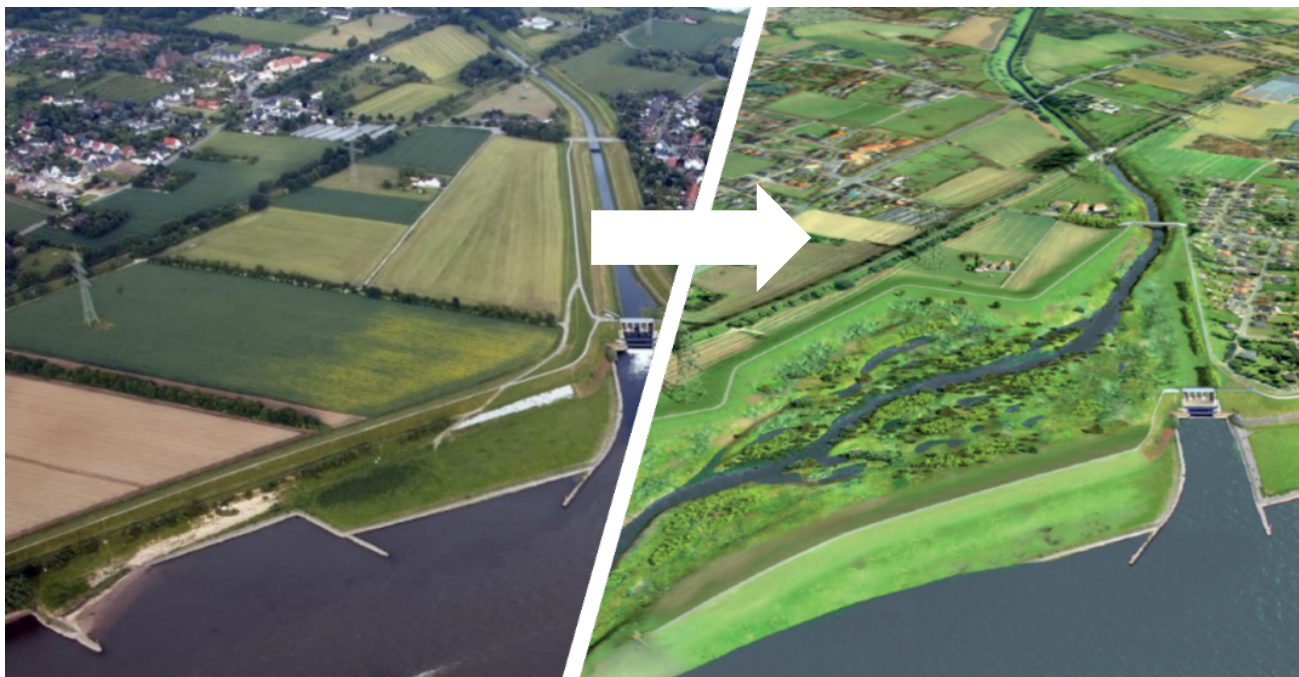
Figure 11: The old estuary of the Emscher with a drop structure of 6 meters to the Rhine (left), newly created Emscher estuary with a 20 ha floodplain (right)
