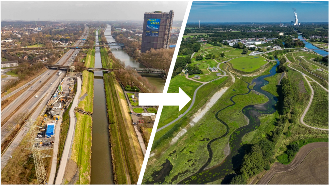
Figure 9: In areas where there is sufficient space, the canalised river can be transformed into a free-flowing Emscher. The Emscher in Oberhausen (left) and the Emscher in Castrop-Rauxel (right) demonstrate the potential of this approach.
